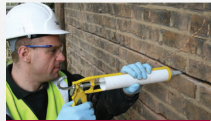
Resin grout installed to receive stainless steel reinforcement
