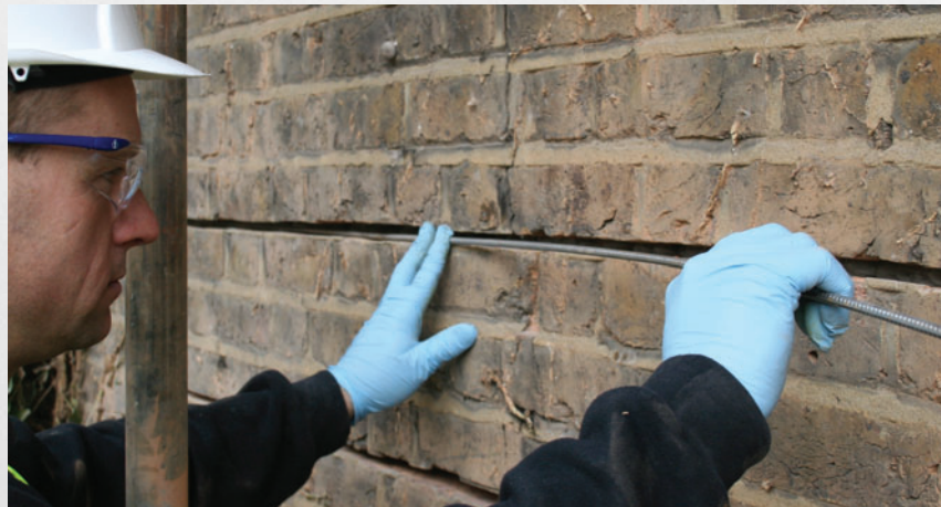
Helical reinforcement being installed in bed joint
