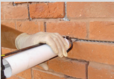
Re-inforcement bedded in resin grout
