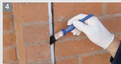
4 Priming prior to installing sealant
