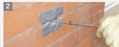
2 Cavity tie installation to restrain brickwork
