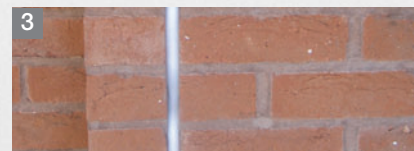
3 With expanded polyethylene foam filler
